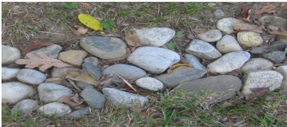
Example of an River Stone Overflow Channel From a Rain Garden
